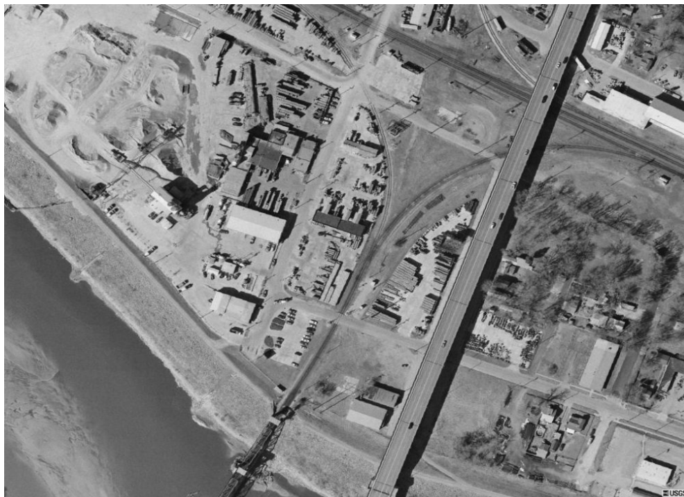
Figure 3. Aerial photograph of a monitored commercial area having unusually high TSS concentrations showing proximity to quarry operation.
